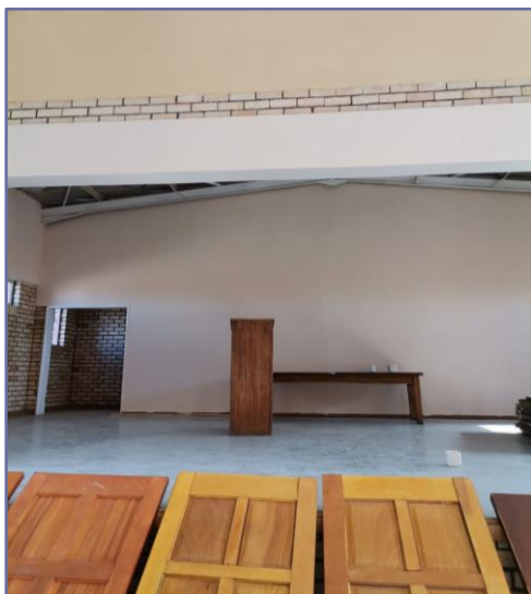
Doors drying after varnish was applied in the foreground and painted walls in the background
